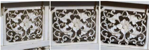
Figure 10: Multiple images used to create a depth map for creating a 3D model.
