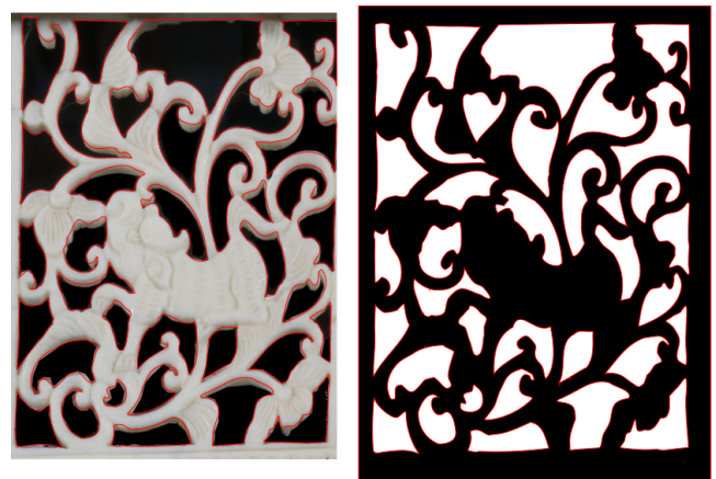
Figure 8: Vectorized window image to generate 3D geometry.
