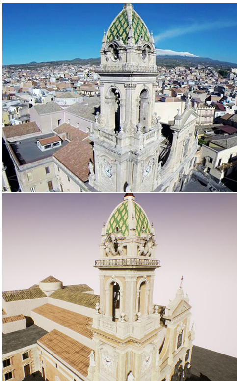
Figure 19: Bell Tower Side by Side between real photo (up) and the final rendering (down)
